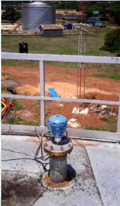
Radar level gauge
